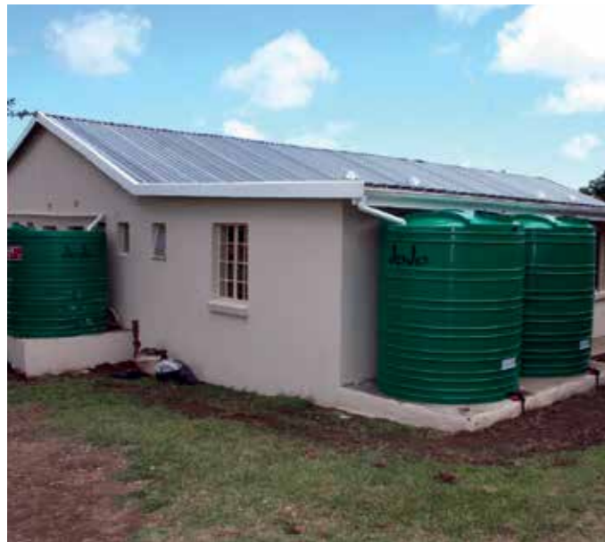
Khula Education, the new school building and tanks.
